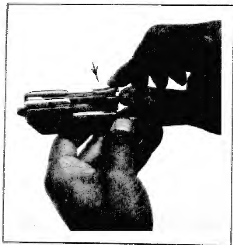
FIGURE 29. REMOVING BOLT
